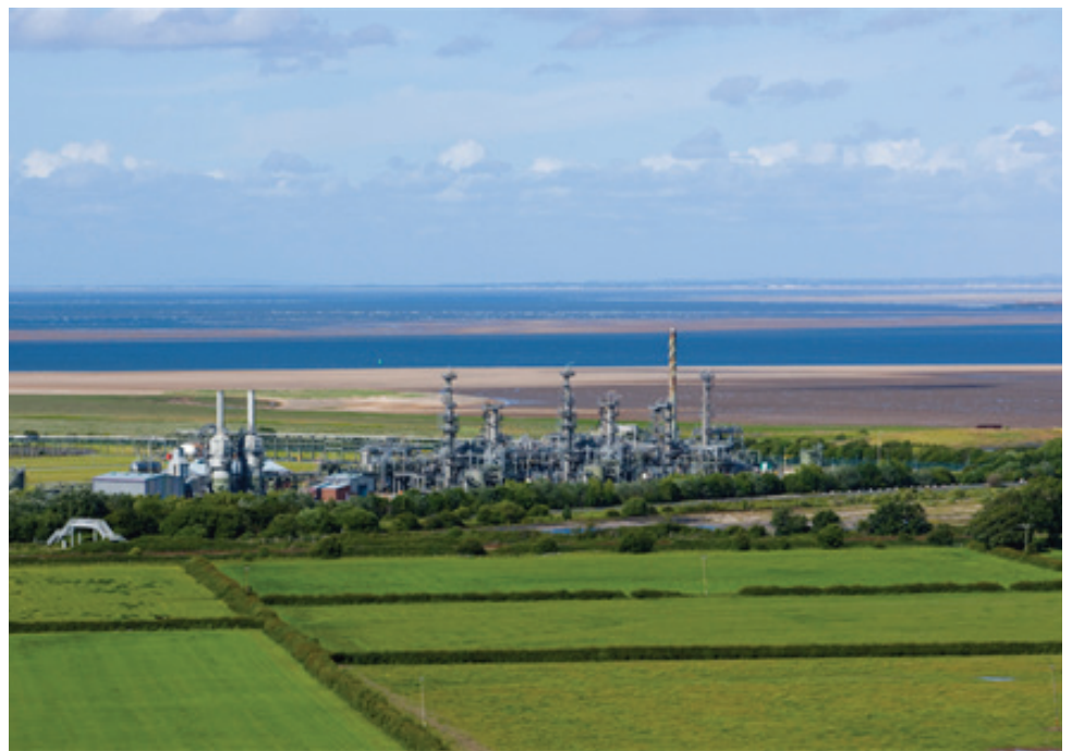
Image 1: Point of Ayr Gas Terminal in Talacre.
