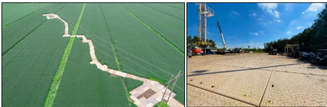
Figure 4.4: Typical temporary matting
