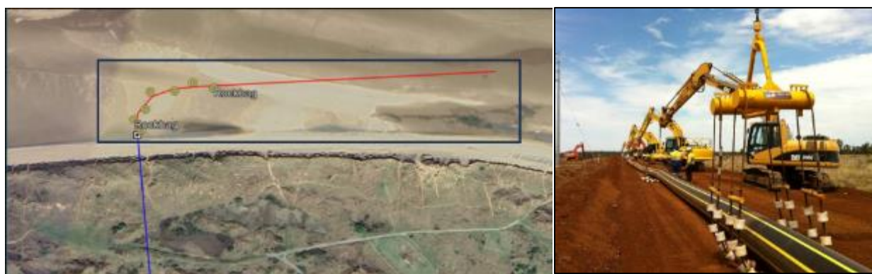
Figure 4.15: Pipe repositioned for pull back
