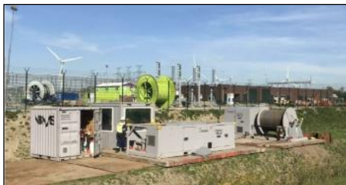
Figure 4.19: Example of typical cable pull winch
