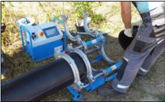
Figure 4.11: Typical pipe welding equipment, storage of pipes and welfare not shown
