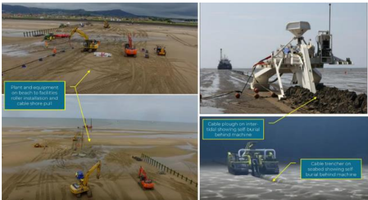
Figure 4.20: Typical plant and equipment for cable installation across inter-tidal like the offshore wind farm cables historically installed between Prestatyn and Rhyl.
