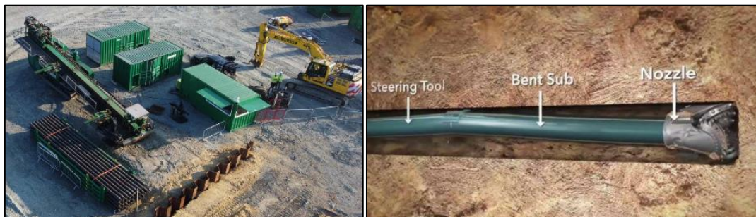
Figure 4.18 Typical Drilling Rig and Pilot Drilling Assembly
