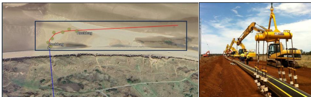
Figure 4.20 Pipe Repositioned for Pull Back
