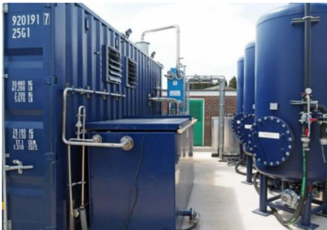
Figure 7.2 Example GAC Filtering System
