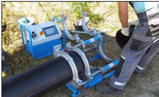
Figure 4.16 Typical Pipe Welding Equipment, Storage of Pipes and Welfare Not Shown
